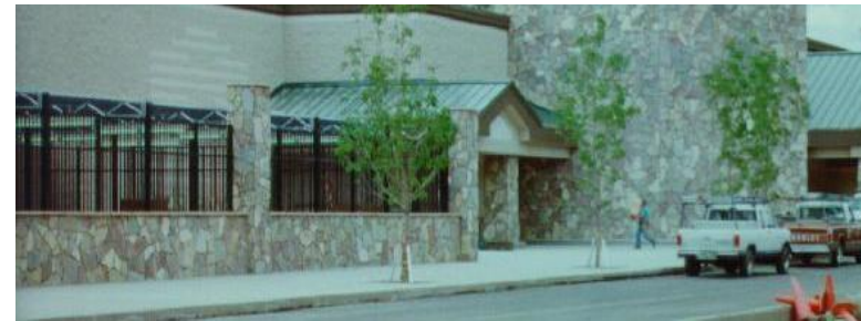
Outdoor Display Screened Behind Front Building Line
