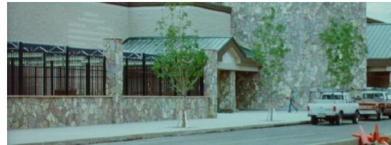
Outdoor Display Screened Behind Front Building Line
