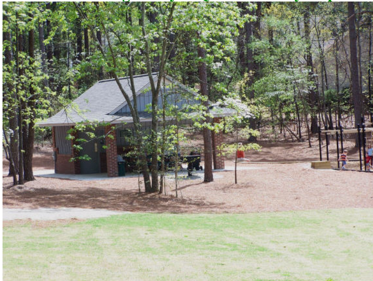
Shelter-Grill-Bathrooms-Water Fountain (even for pets)
